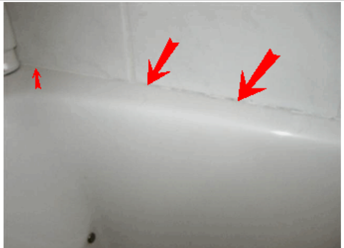
Seal between jet tub and walls
